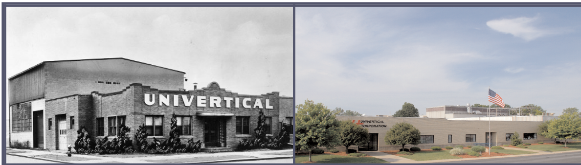
Then and now: Univertical’s Angola, Ind., plant, expanded in 1996, provides: 80,000 square feet for anode manufacturing; 20,000 square feet for chemical manufacturing; 40,000 square feet for warehousing; 5,000 square feet for machine shop and maintenance; and 10,000 square feet for engineering and administration.
